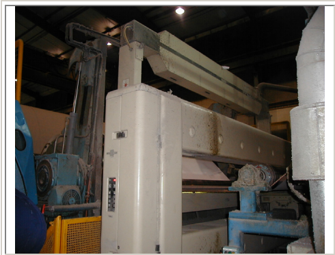
South East Asian Installation
