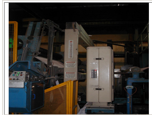
South East Asian Installation
