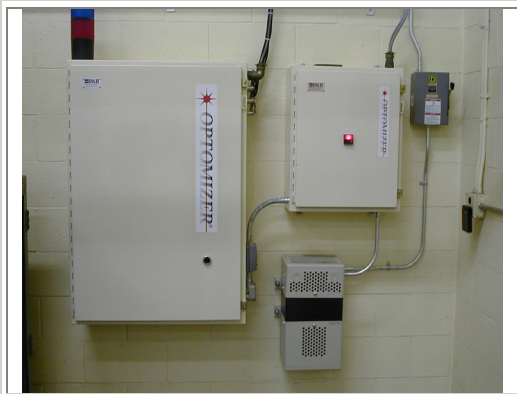
Electronic Control Stations
